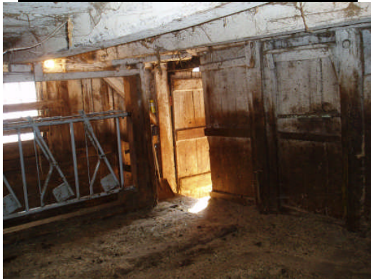
The Tyrrell Barn on 20 Mile Stream Road
